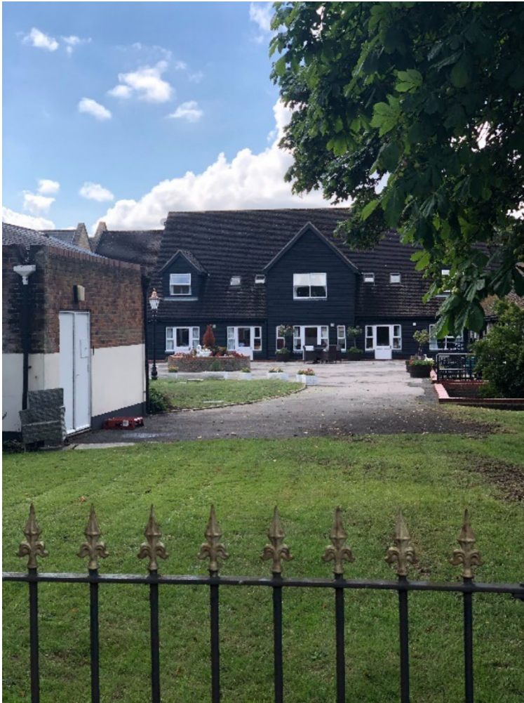
View of external secure hard-surfaced area from perimeter fence
